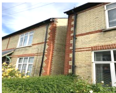
Brickwork detailing, Fulbrooke Road
