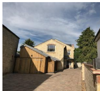
New build in back garden
